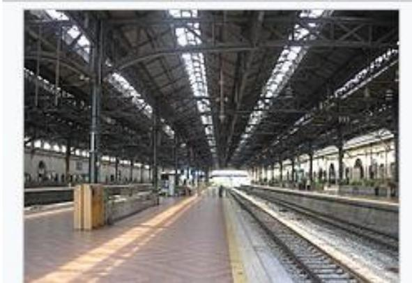
The original platforms of the station (pictured before 2009 platform renovations) retain older architectural elements, such as the large steel-framed pitched-roofed train shed.
