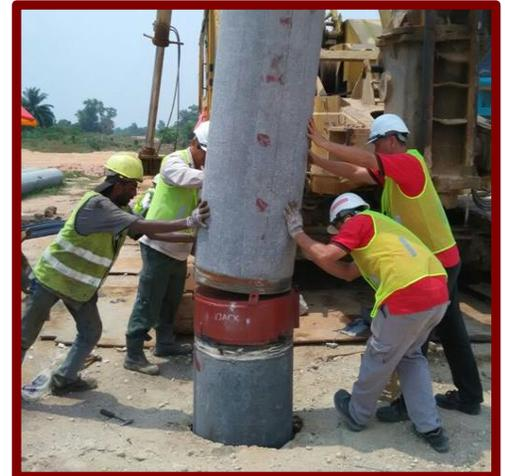
**YJACK Technology Sdn Bhd is an independent, competent and professional company offering pile testing services. Our world patented innovative pile testing method, YJACK Bi-directional Pile Load Test, caters for a broad range of loading capacities and pile sizes that meet the industry's requirements, locally and globally.**
